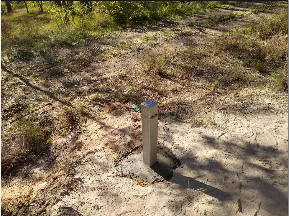
Figure 6: Typical Well installation on site
